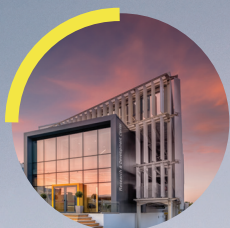
New state-of-the-art Research & Development Center of 2,500 m 2 with laboratories of high technological standards
